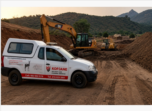
Construction site security
